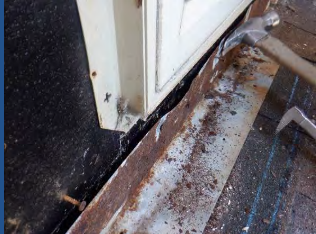
Omitted SAF and sealant; improper fastening
