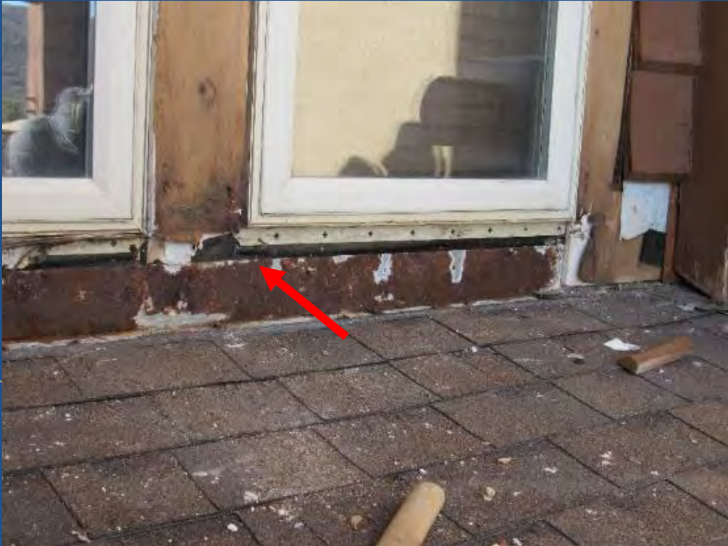
Improper and deteriorating flashing
