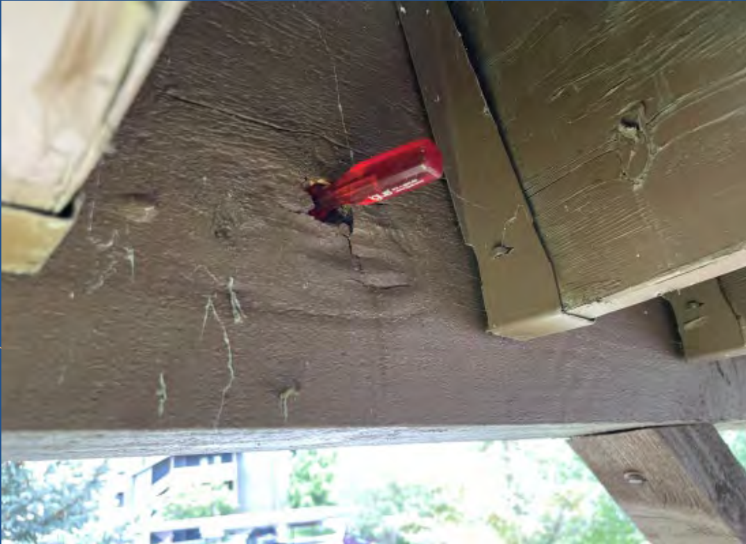
Decayed deck beams (10-20%)
