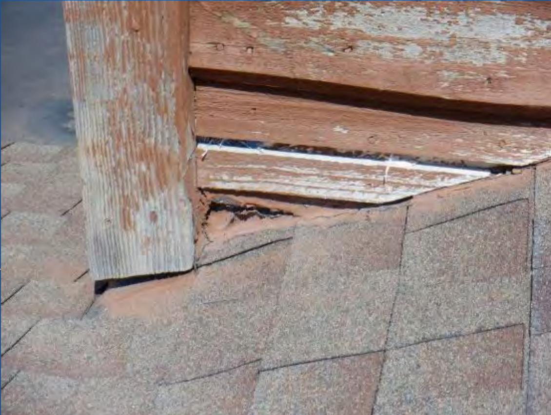
Improper roof-to-wall integration
