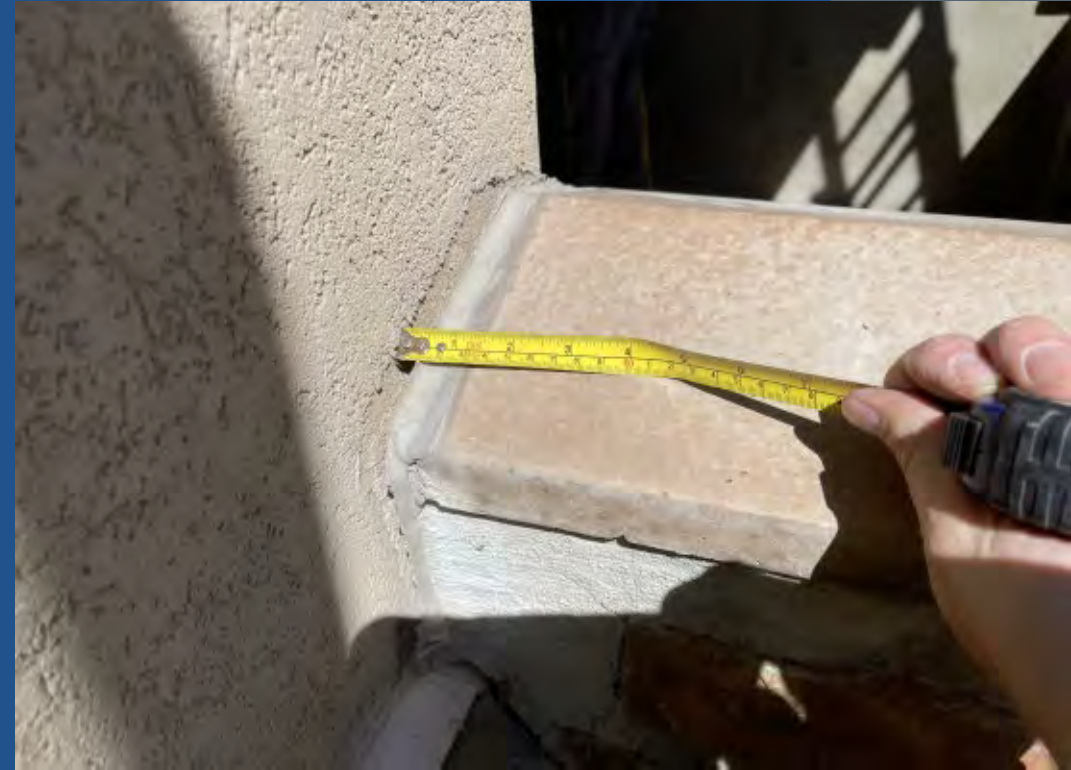
Lower floor patio wall pulling away from building due to foundation settling
