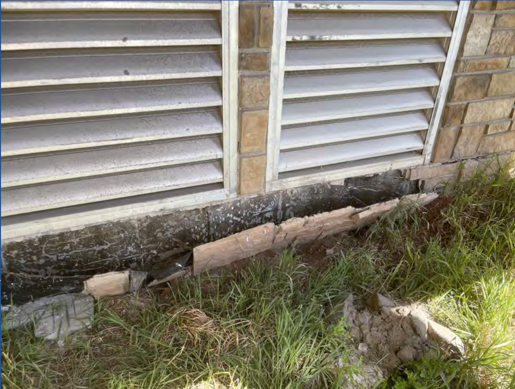
Manufactured stone veneer assembly failure
