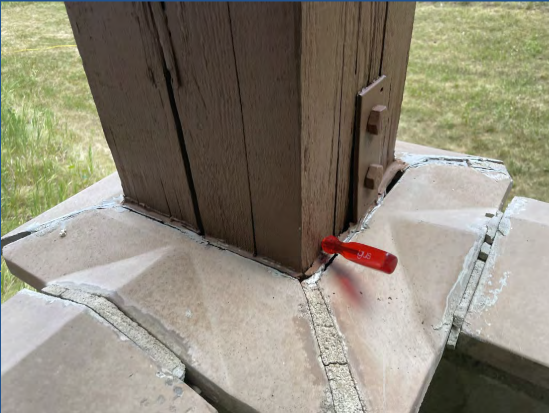
Wood decay at base of column
