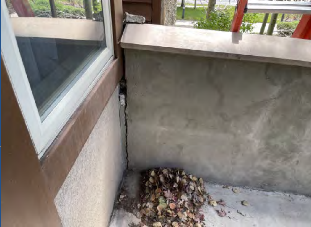
Lower floor patio wall pulling away from building due to foundation settling
