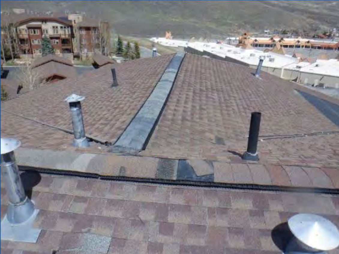
Granule loss and shingle damage
