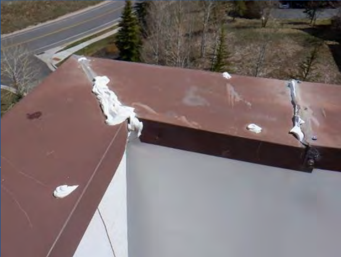
Sealant dependent coping (and improper sealant).
