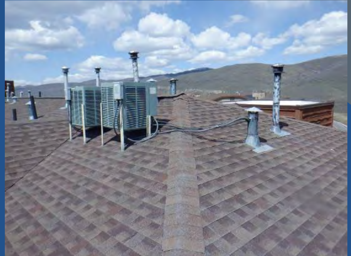
Improper mounting penetrations at rooftop mechanical equipment.
