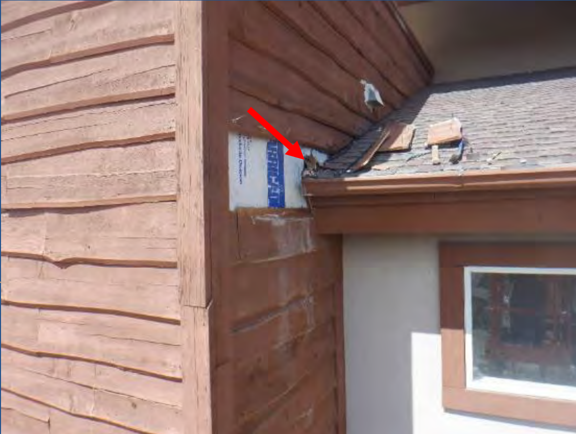
Improper diverter resulting in water intrusion at walls
