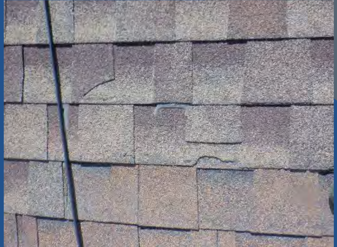
Granule loss and shingle damage
