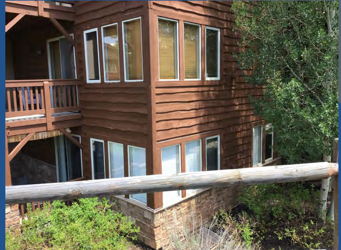
High maintenance horizontal siding; prone to cracking, cupping and finish deterioration
