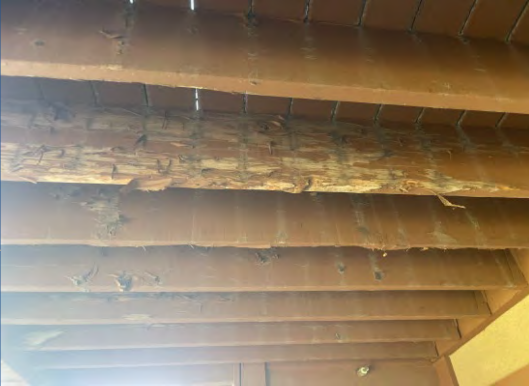
Decayed deck joists (35% +/-)
