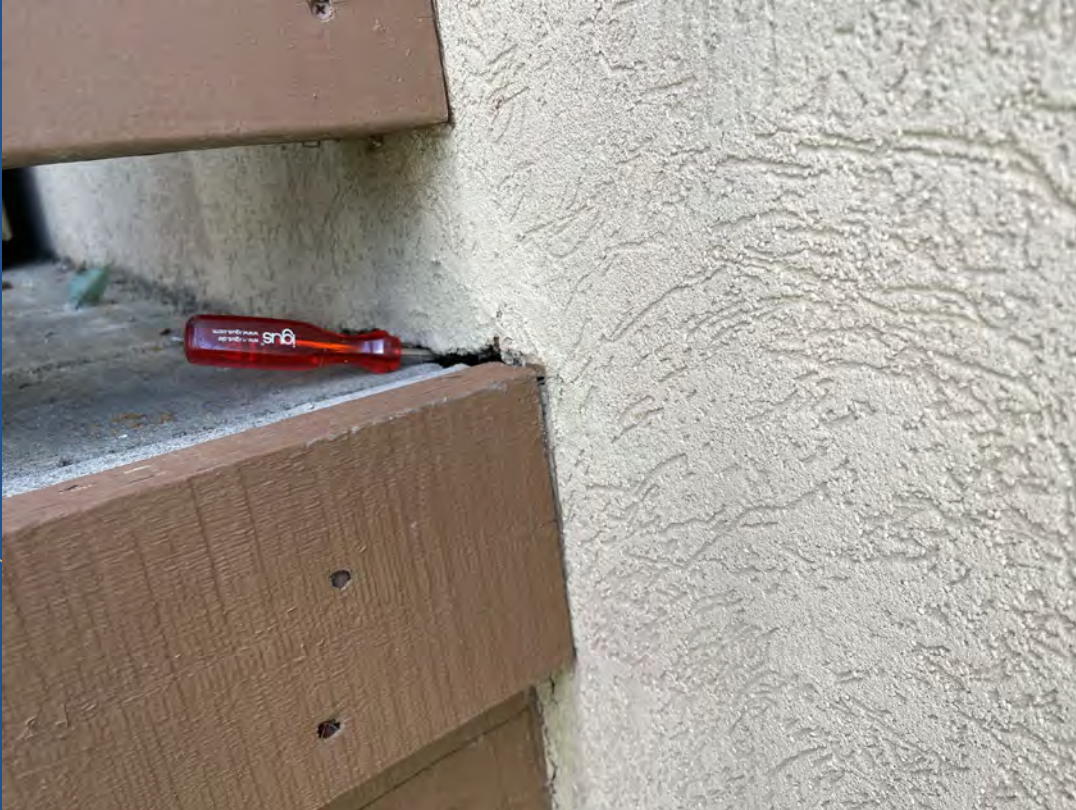
Open void into wall cavity at deck to wall locations
