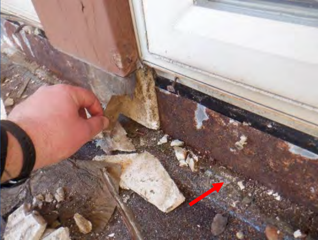
Water damaged WRB and sheathing
